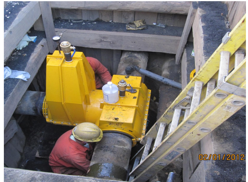
Joint Encapsulation completed by Maintenance and Repair
