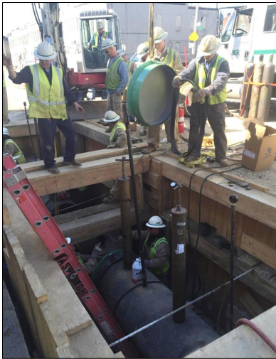
Abandonment of 30" Cast Iron main (BOP: Edmondson)
