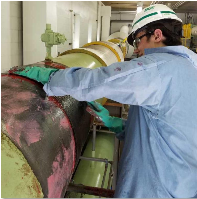
Installing Black Diamond Carbon Fiber Wrap
