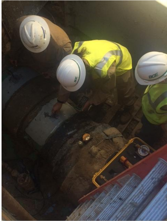
Inspecting Transmission Pipe
